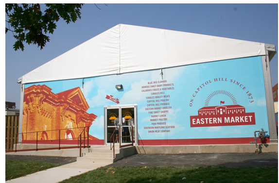
Eastern Market Temporary Building
