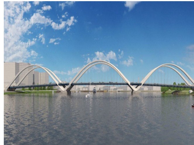
Credit: Courtesy of South Capital Bridge Builders and Walsh Group
